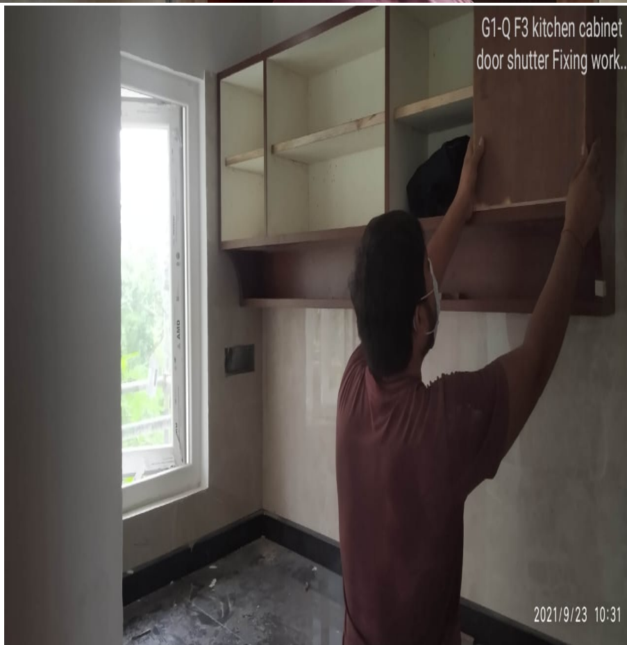
G1-Q F6 kitchen cabinet shutter's fixing work...
