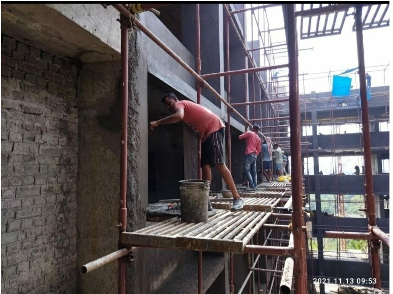
Sarayu- Outer plastering work in progress.
